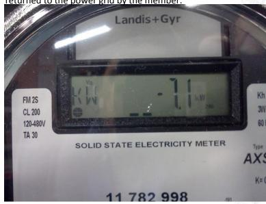
The meter indicates "KW" on the left hand side of the LCD display to provide an immediate indication of how much power is being delivered to the member or excess power being supplied by the member to the power grid. When energy is being provided to the member from the power grid the "KW" value will be positive. When energy is being returned to the power grid from the member the "KW" value will be negative.
