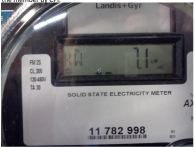
"KW" display indicating 7100 Watts of excess power being returned to the power grid by the member.
