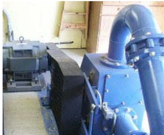
*Belt drive coupling between turbine and generator.*
